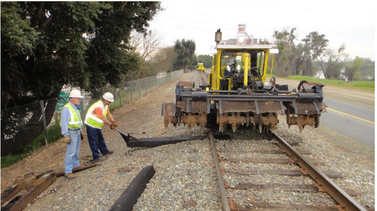
Heather in the scarifier-inserter pulls in a new tie guided by Mike M. and John.
