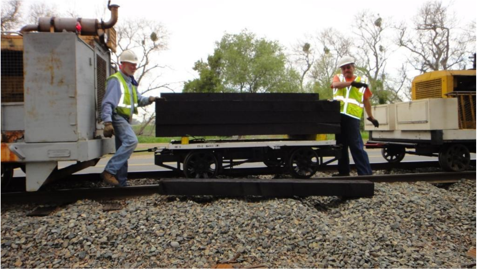
Mike M. and John drop ties off the flatcar next to empty cribs.
