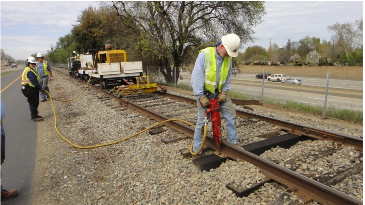
Heather guides the air hose from the compressor while Mike M. uses the pneumatic spiker to drive spikes.
