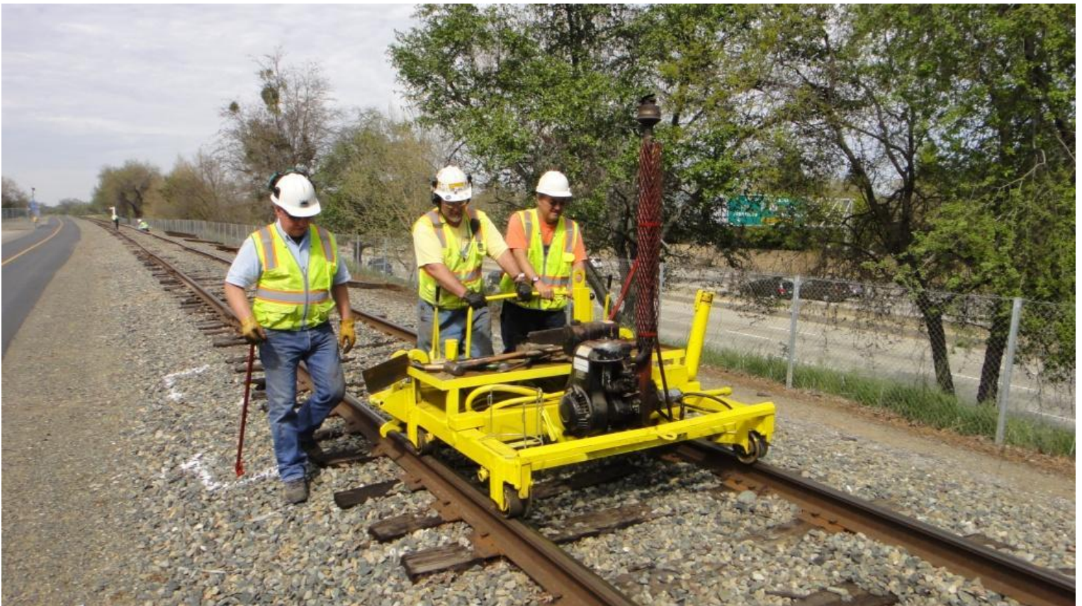
The rail-lifter finally arrives after being delayed by the UP's computer problems. Ed, Mike F., and John get it into position.
