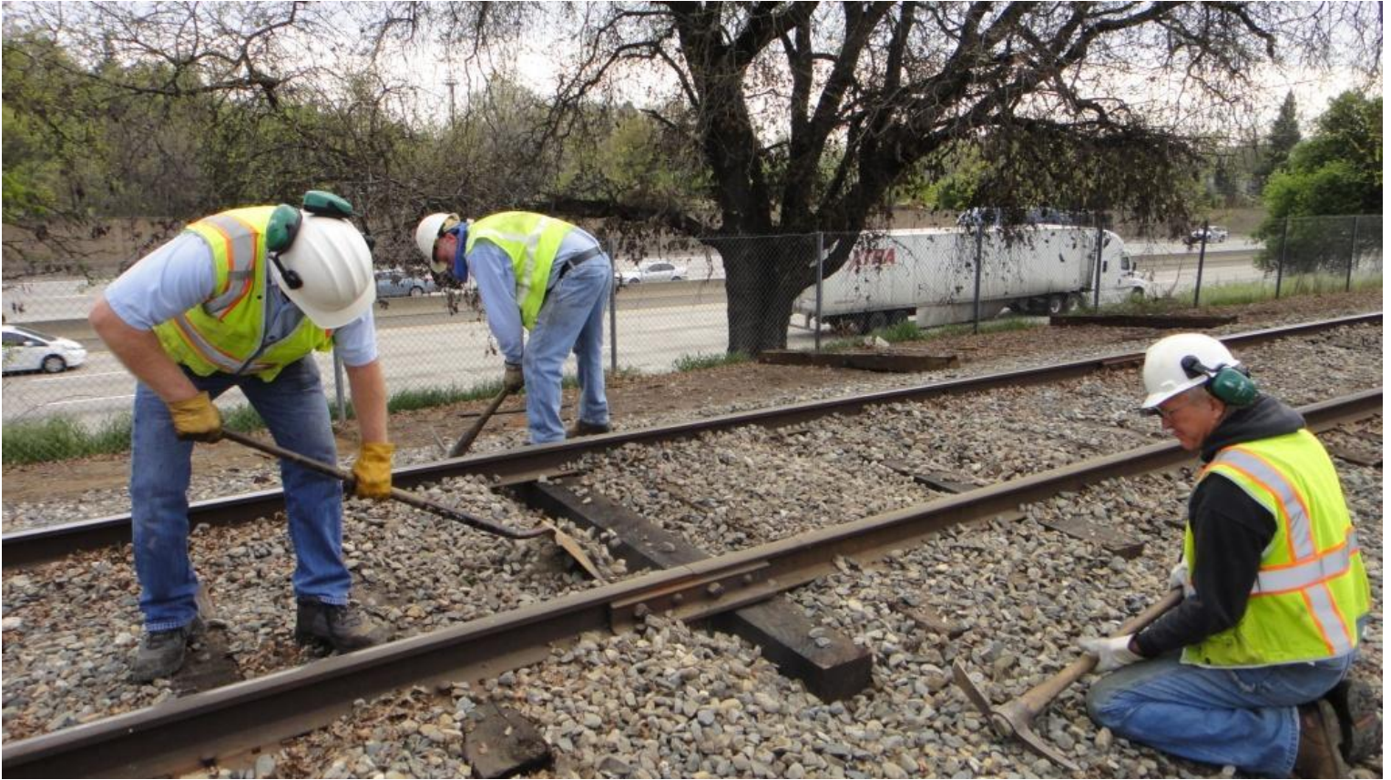
Ed, Mike M., and Steve N. fill in ballast around the newly inserted tie in preparation for tamping.
