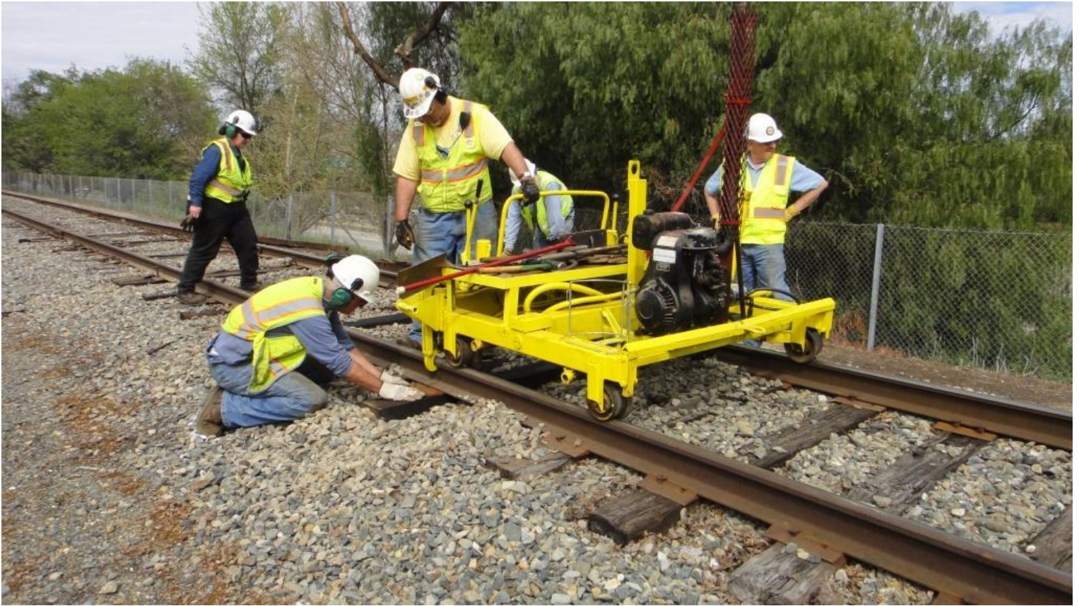
Mike F.'s skillful touch raises the rail just enough for Steve N. to insert a tie-plate.
