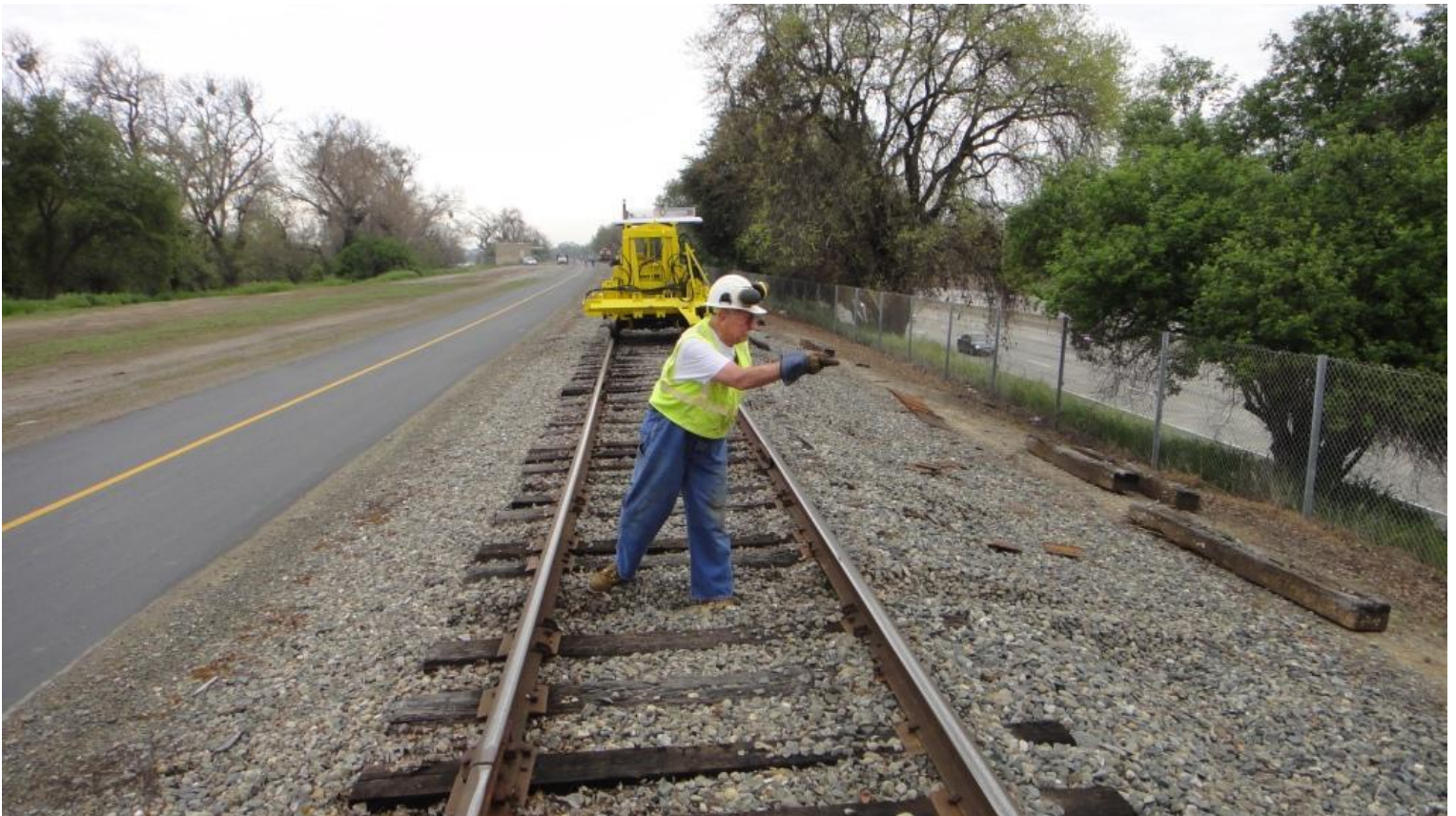
Meanwhile, down at the worksite, Clem locates and tosses tie-plates out of the way so that they wouldn't get buried by the scarifier.
